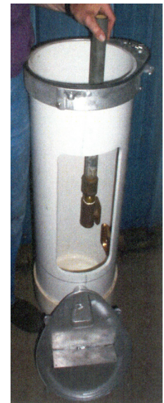
PVC Casing with Pitless Adapter apart
